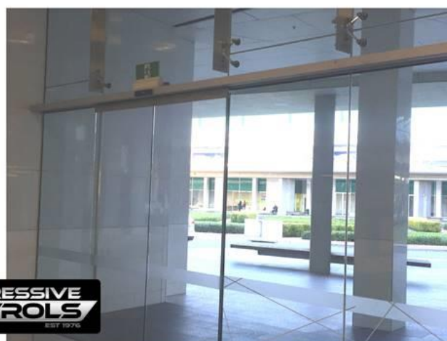
Canberra International Airport internal photo of GEZE 70mm SL drive mounted directly to glass.
